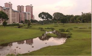
This bioswale, in an urban park setting, is allowed to fill up during heavy rain water events and drain slowly after. It has become an amenity within the park and has significantly increased the amount of biodiversity within the park. Residential and public green spaces should be designed to deliver multiple benefits like this park achieves.
