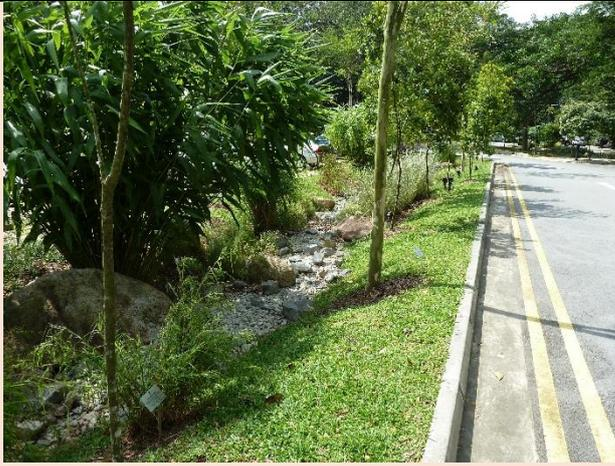
Bioswales can be used in urban areas to manage and treat rainwater runoff from roads, car parks and other hard surfaces. They allow the water to drain slowly into the ground. Vegetation helps treat the water and add biodiversity value & visual interest.
