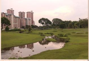
This bioswale, in an urban park setting, is allowed to fill up during heavy rain water events and drain slowly after. It has become an amenity within the park and has significantly increased the amount of biodiversity within the park. Residential and public green spaces should be designed to deliver multiple benefits like this park achieves.
