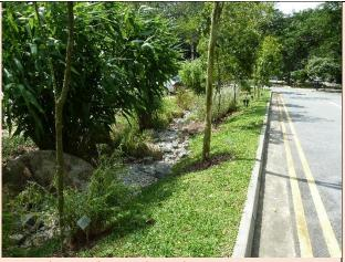
Bioswales can be used in urban areas to manage and treat rainwater runoff from roads, car parks and other hard surfaces. They allow the water to drain slowly into the ground. Vegetation helps treat the water and add biodiversity value & visual interest.
