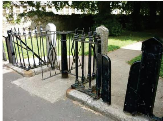
Fig.48 View of cast iron gate and granite posts to the Laurels.
