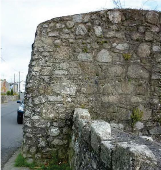
Fig.67 Detail of restored stonework at Carlow Gate.
