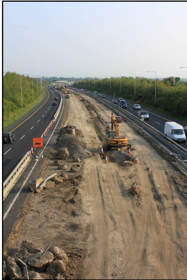
Plate 11.2: M1 Widening project under construction
