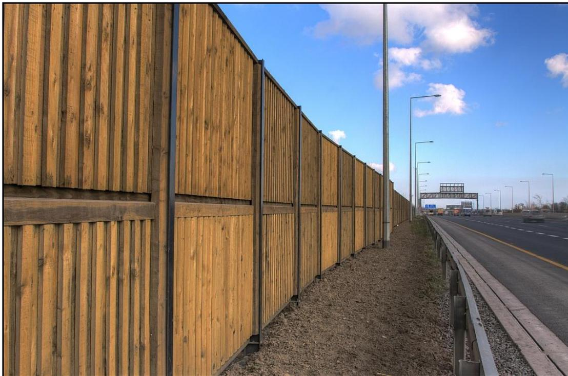
**Plate 4.12: Example of Noise Barrier at the back of verge (M50 Dublin)**
