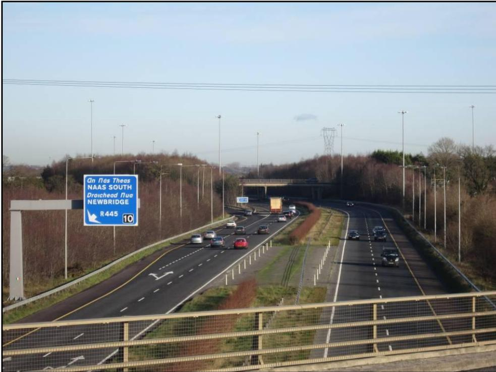
**Plate 4.3** Existing two lane M7 with wide grass median, looking north east toward Newhall Interchange
