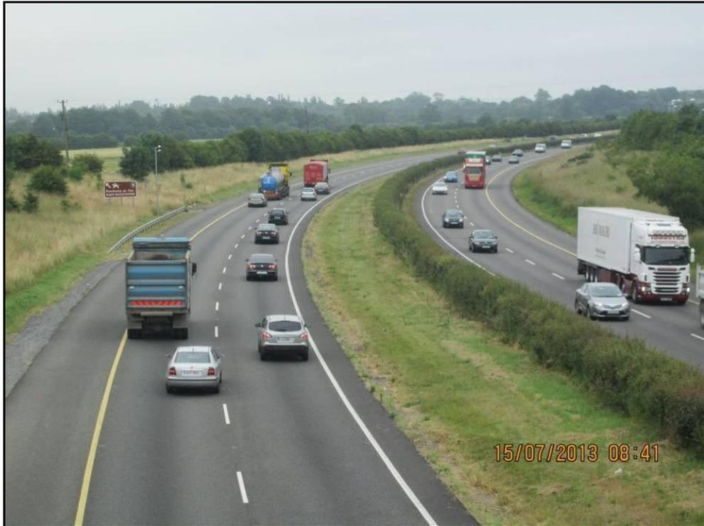
**Plate 4.5** Existing two lane M7 with wide grass median, looking north east from the R407 overbridge
