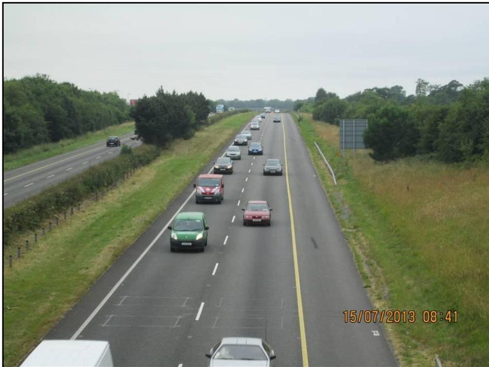
**Plate 4.6** Existing two lane M7 with wide grass median, looking south west from the R407 overbridge
