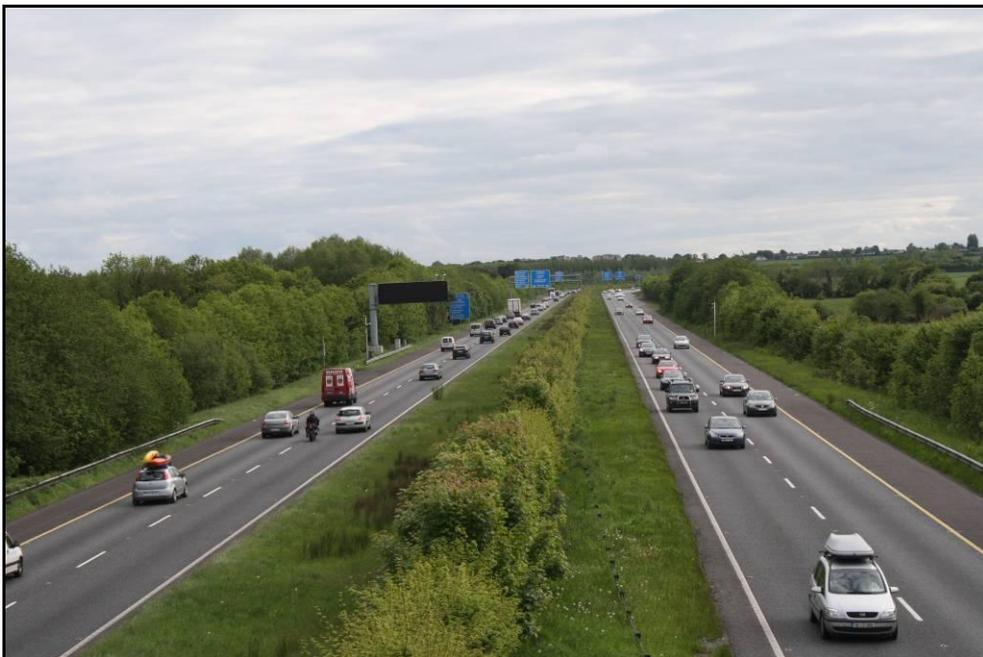
**Plate 4.2** Existing two lane M7 with wide grass median and planted embankments at Lewistown
