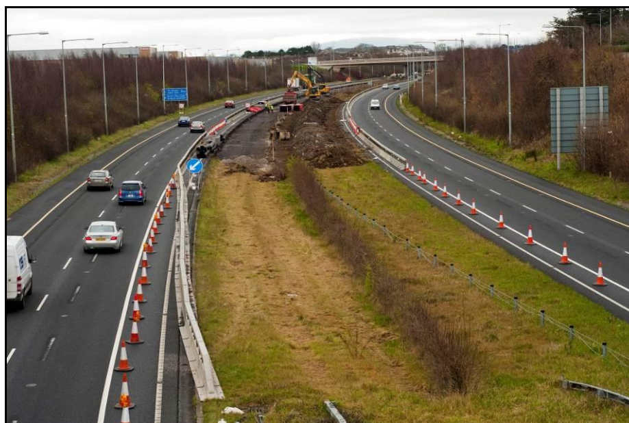
Plate 5.2: M1 Widening under construction
