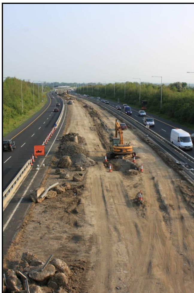
Plate 12.2: M1 Widening project under construction
