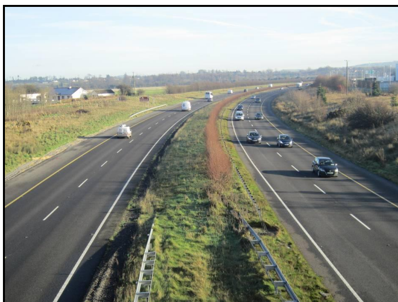
Plate 12.1: Typical stretch of the M7 highlighting width of central median
