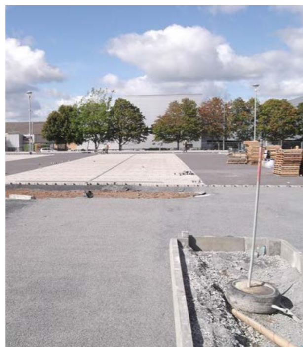
Image below: Landscape construction 1.
