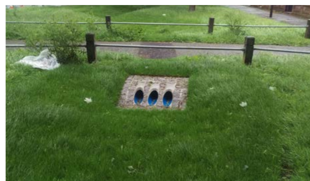
Image above: Concrete pipe surround has been used here to provide minimal cover for a driveway crossing
