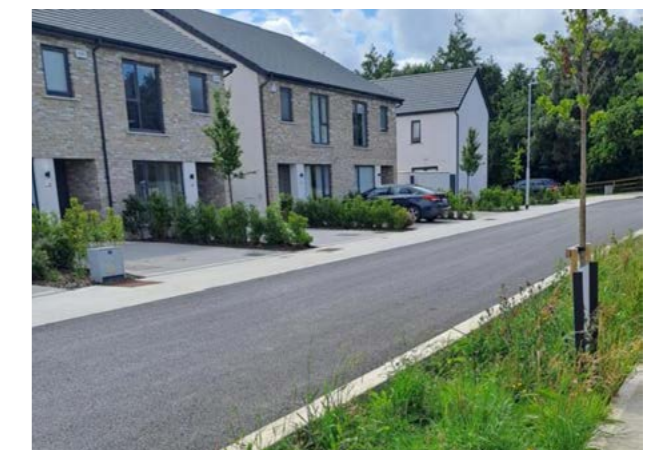
Image above: Collection of rainfall runoff through openings in kerb into a linear rain garden. Residential development, Leixlip
