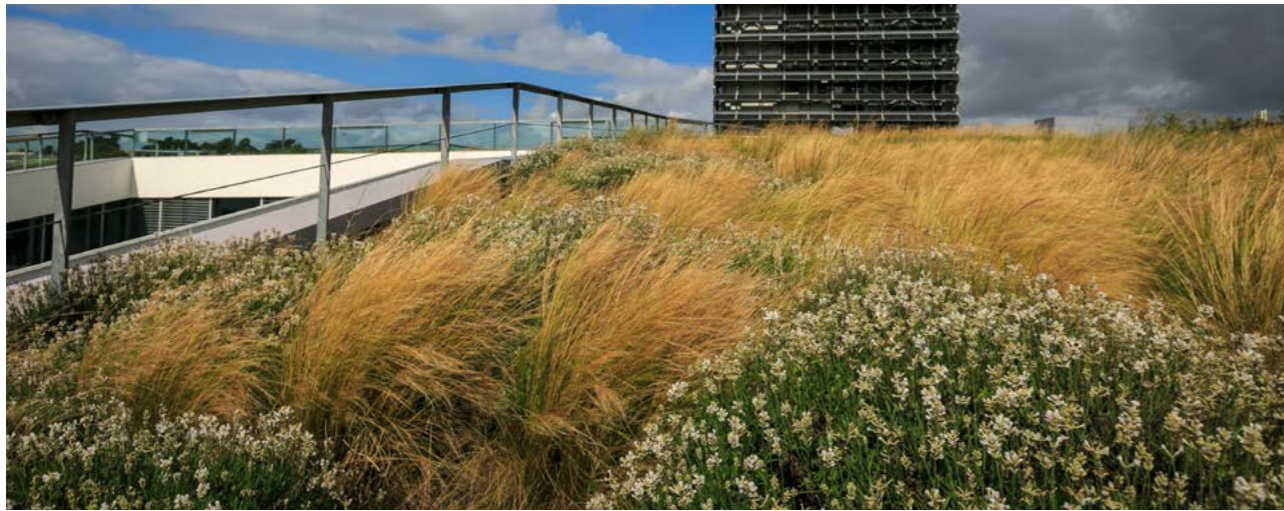
Image above: Green roof on the Bord Gaís Networks building, Finglas
