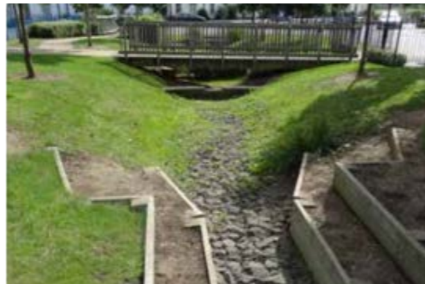
Image below: Demonstrates impact of erosion
