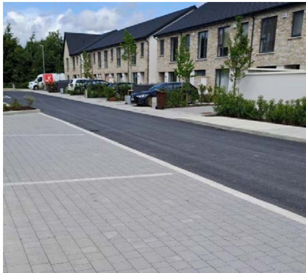
Image above: Strategic Housing Development Harpur Lane, Leixlip, Co.Kildare - Permeable pavement managing runoff at source.
