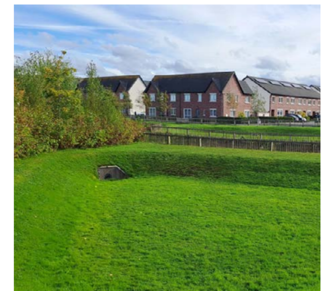
Image above: Detention Basin in public open space - Elsmore Naas
