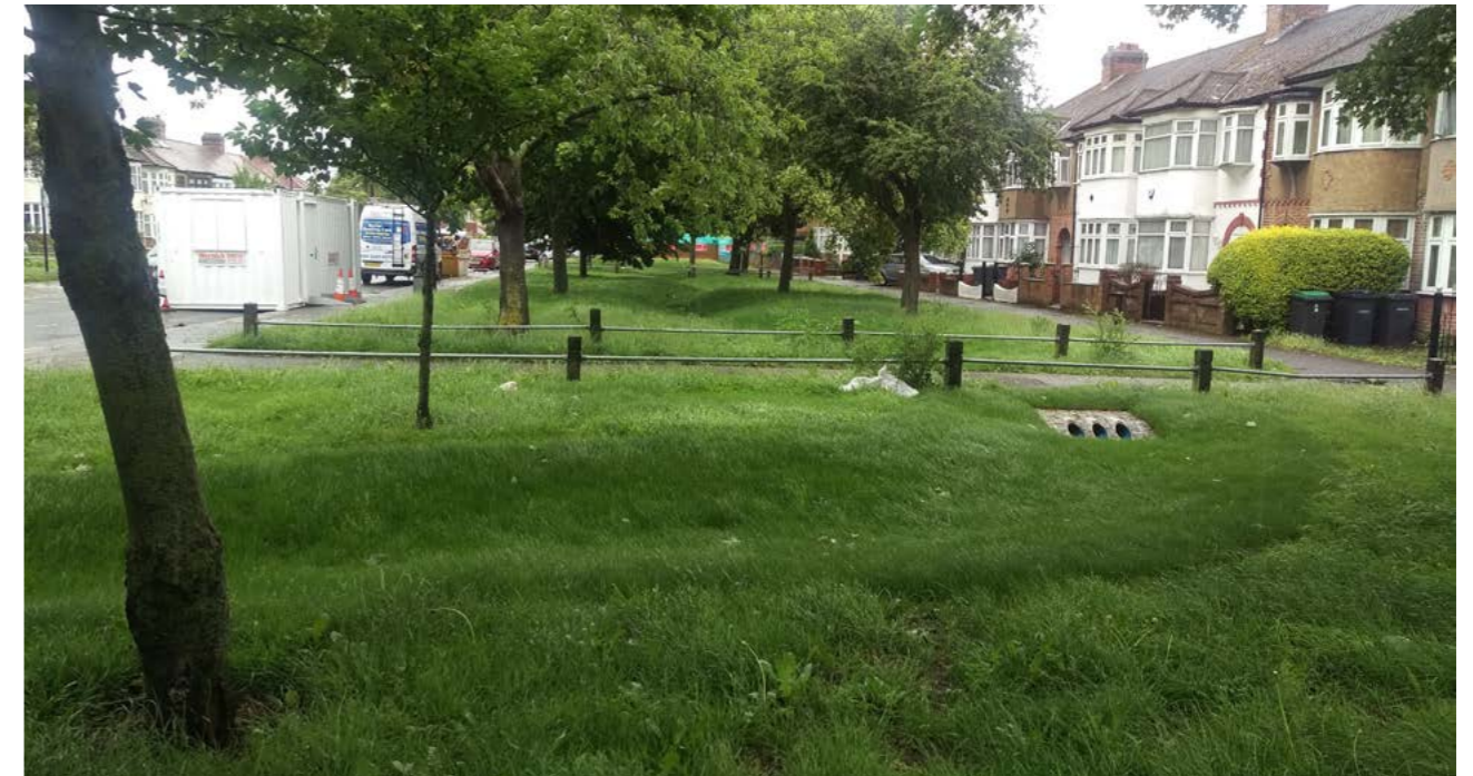
Image above: Shows shallow short piped connection under a driveway allowing the swale to remain shallow downslope.
