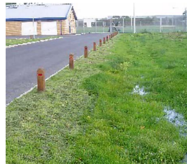
Image above: Low risk access road with 1.2m wide filter strip source control and conveyance swale.
