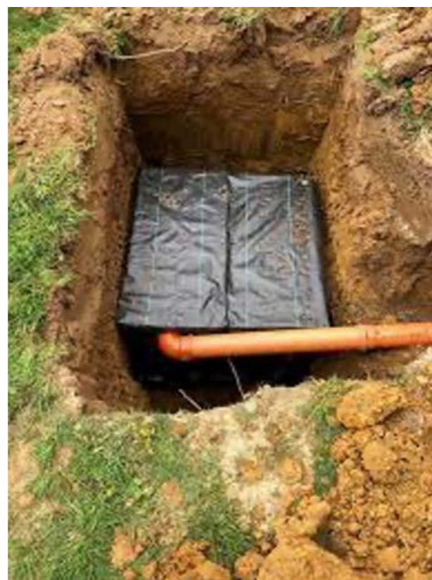
Image above: Example soakaway feature during construction
