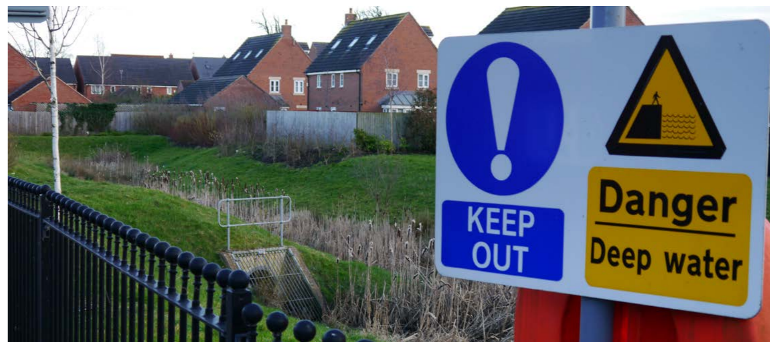
Image below: This project failed to adequately consider health and safety when designing attenuation features into a residential pocket park. There is now no public access allowed. There should be no need for such measures if properly designed.
