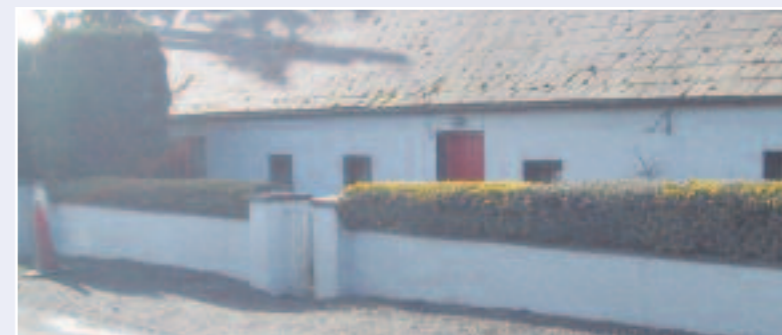
Traditional cottage and doorway, Nurney
