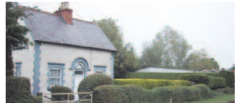
Gable view of County Council cottage
