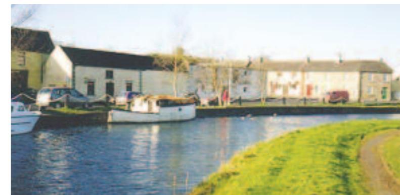
Robertstown - canal-side from East
