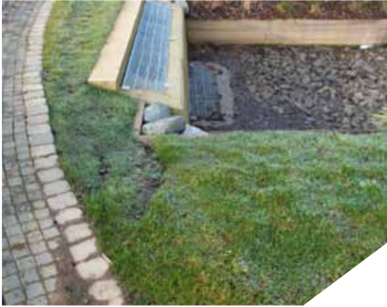
Figure 15.14 Swales at Upton, Northhampton, UK
