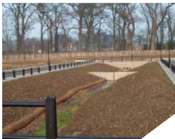
Figure 15.13 Swales at Upton, Northhampton, UK
