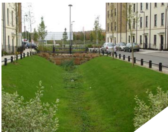
Figure 15.12 Swales at Upton, Northhampton, UK
