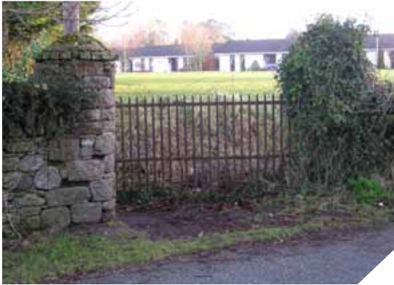
Figure 16.43 Stone wall, pillars and gate, Naas
