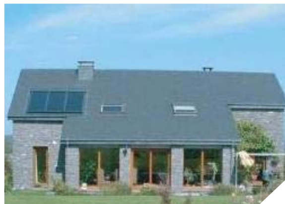
Figure 16.47 Image of roof solar panel
