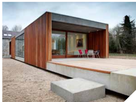
Figure 16.48a Refurbishment and Extension. Ballymahon House. ODOS Architects
