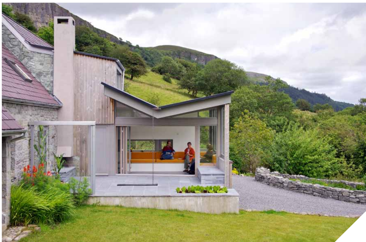
Figure 16.11 Landscape room, Co. Sligo. LID Architects
