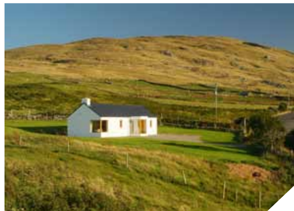
Figure 16.23 Contemporary house design based on traditional narrow plan. Louisburgh, Co. Mayo. Cox Power Architects
