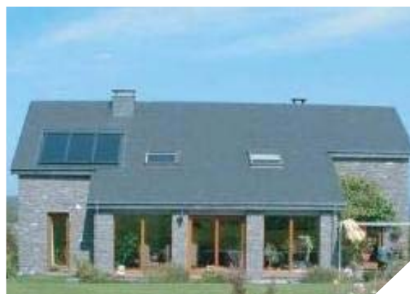
Figure 16.47 Image of roof solar panel
