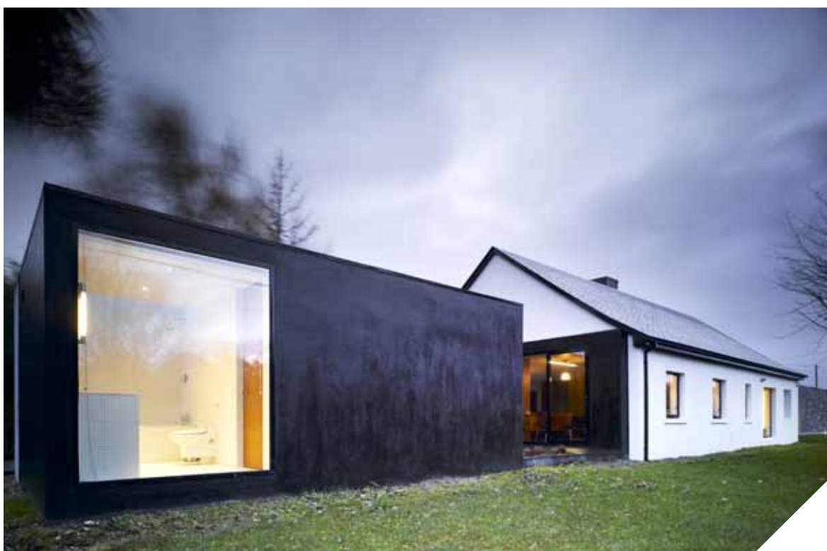
Figure 16.50 Extension to side of house. Glengowla, Co. Galway. Boyer Kennihan Architects.
