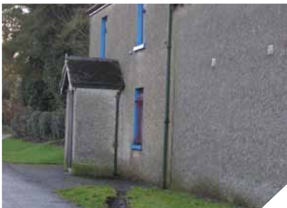
Figure 16.37 Traditional House with Porch, Naas
