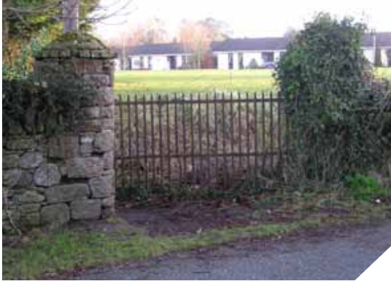
Figure 16.43 Stone wall, pillars and gate, Naas
