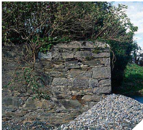
Figure 16.41 Image of traditional stone wall at Devoy Barracks, Co. Kildare
