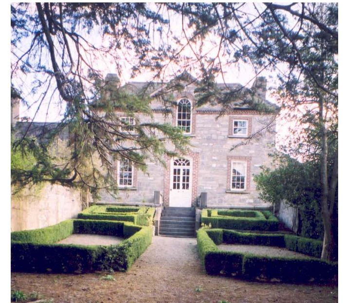
Fig. 1.6 Kildought House—an architecturally important house set back from the main street with fine rear garden onto the river
