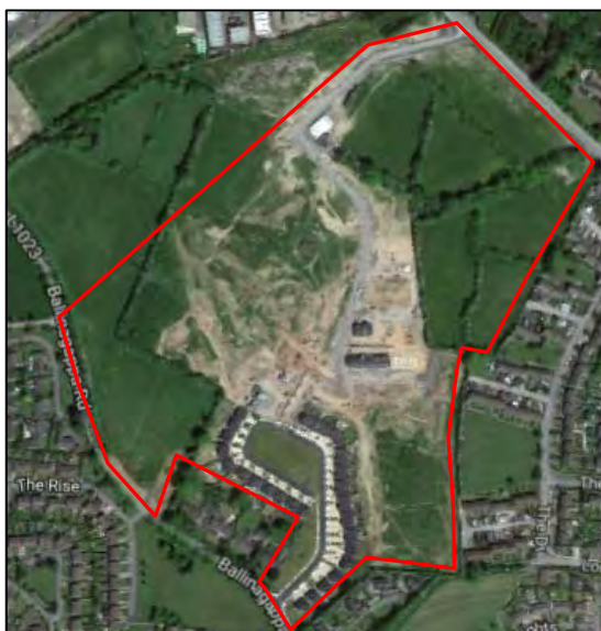
Figure 12.4 a) KDA 3 Aerial View
