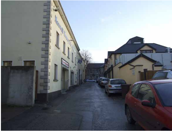
Lack of active frontages and poor public realm along Kelly's Lane
