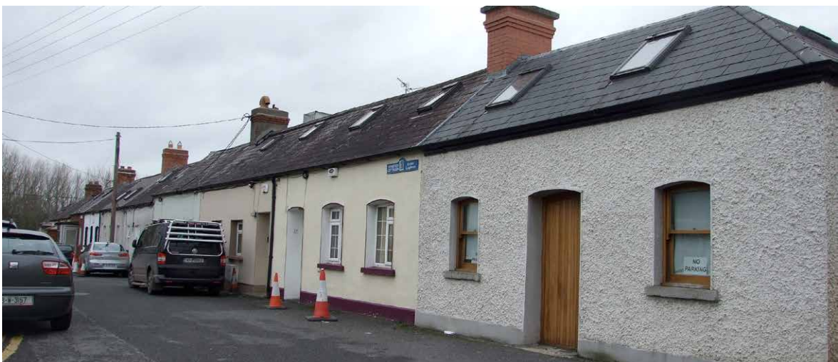
View of labourer's cottages
