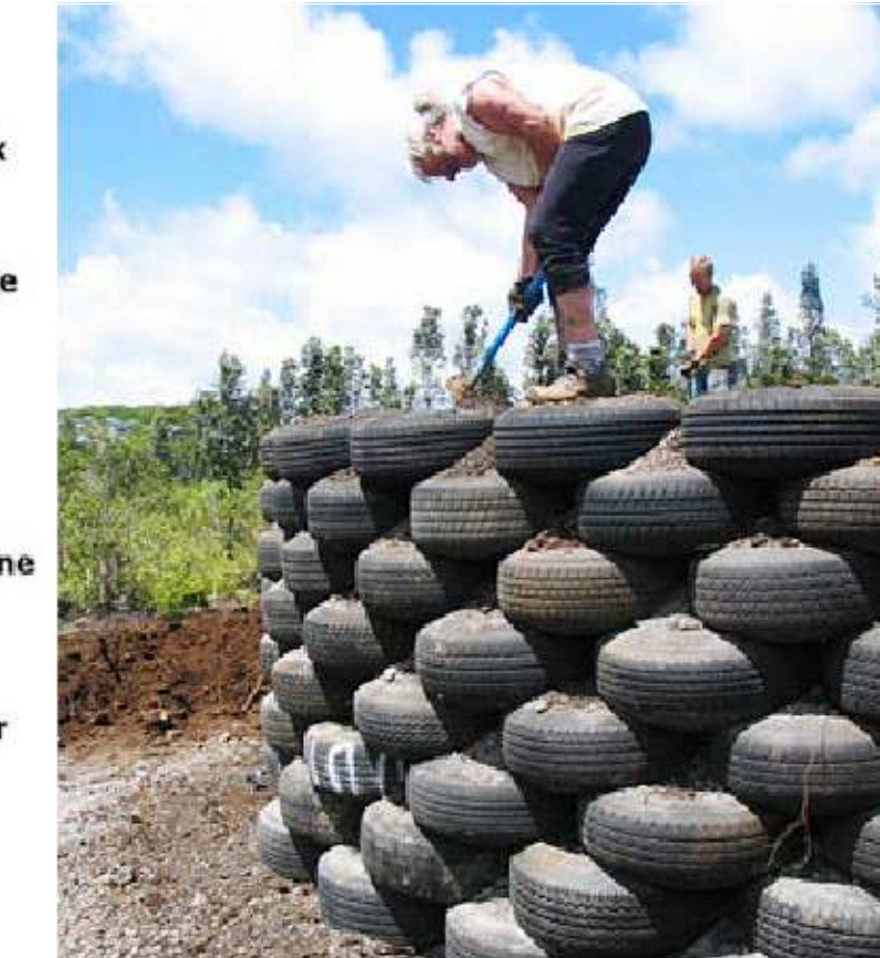
PROPOSED TYRE RETAINING WALL
