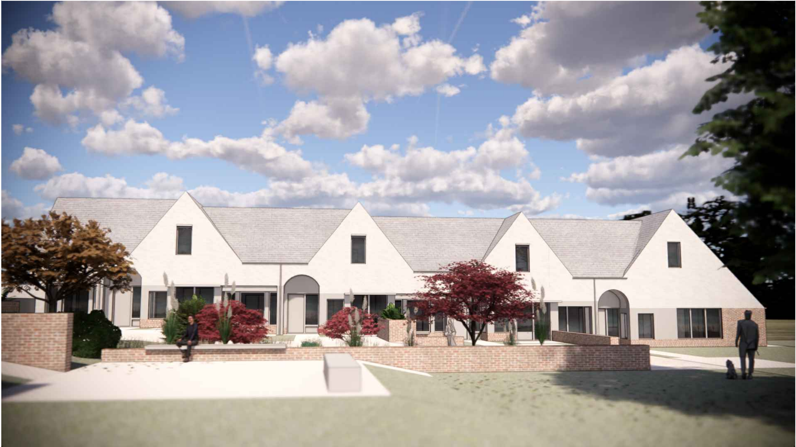
1 VIEW FROM BUILDING B NTS@A3
