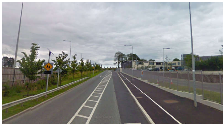
Figure 4-7: Naas to Kill Section 4: View Eastbound Approaching Scoil Bhríde
