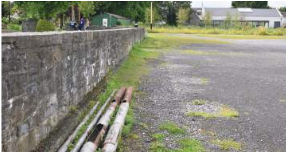
Stone built retaining wall with 0.7M level change
