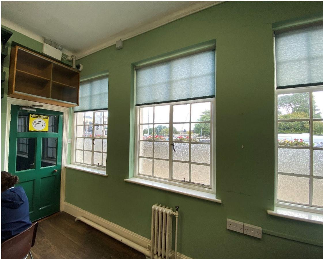
Figure 41: Original library reading room, with simple coved cornice, panelled doors, moulded architraves, cast-iron radiators with surface-run pipework. Smooth plaster walls with paint finish.
