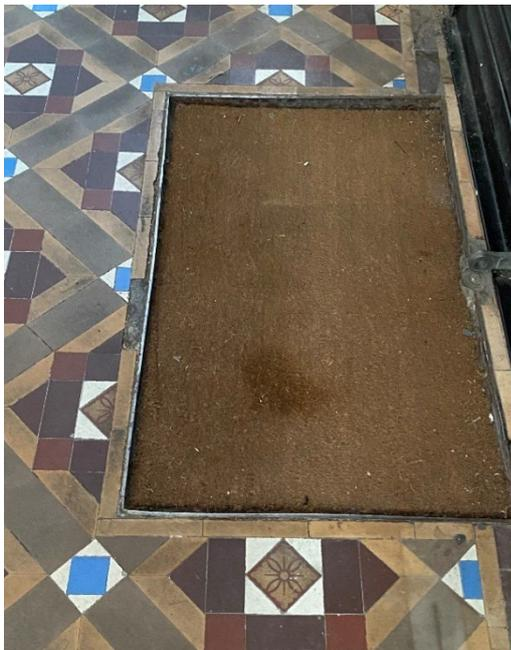
Figure 67: Encaustic patterned floor tiles with sunken mat well at main entrance
