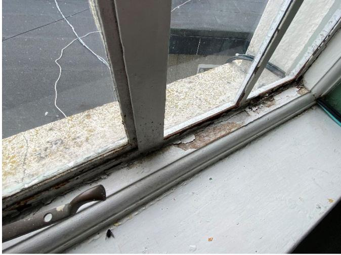
Figure 46: Detail of steel windows which are housed in timber moulded sub-frames with timber window boards
