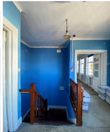
Figure 56: First floor landing with simple coved ceilings and early light fittings still in place
