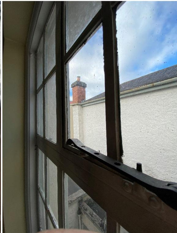
Figure 51: Windows have T-bar sections; all astragals overlap rather than a splice joint.
