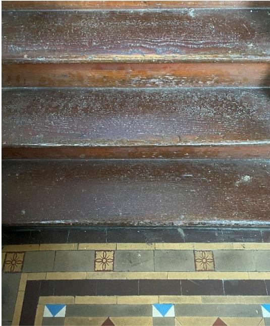
Figure 65: Pine timber treads and risers to main staircase
