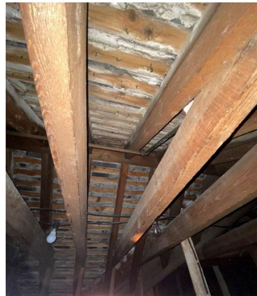
Figure 63: Water staining at wall plate level beneath parapet gutter boarding
