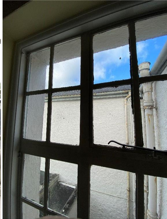
Figure 49: Detail of steel window sitting in timber sub frame Figure 50: Detail of pin stay mechanism
