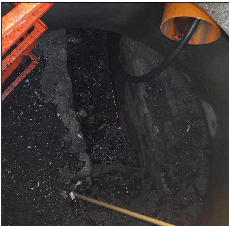
**Figure 4: Manhole Opening at Historic Brick Sewer**
