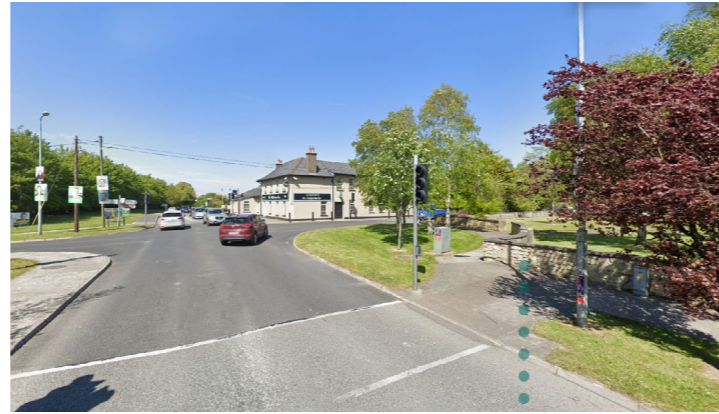
Above: Athgarvan Crossroads Photo of Athgarvan Crossroads as existing. The public space is dominated by the car.
