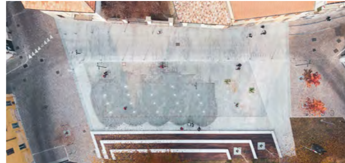
Example of a shared space, raised table area. Source: Landzine.com. Photo by: Daniele Pavesi. Project: Desio, Italy. Designer:Openspaces
