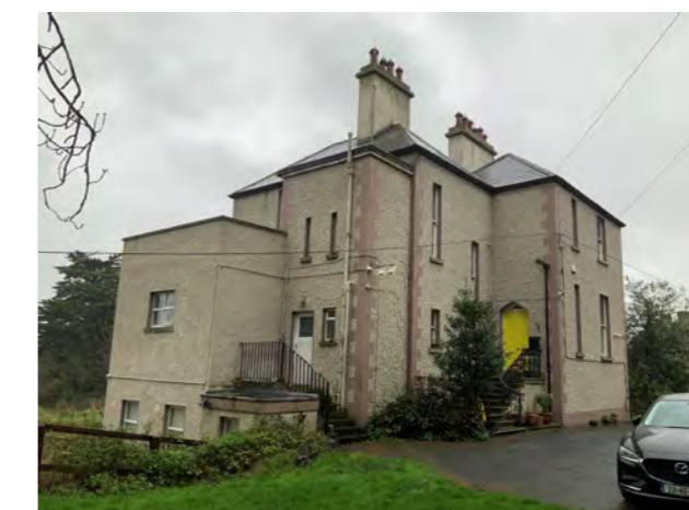
View towards Parochial House from the north.
