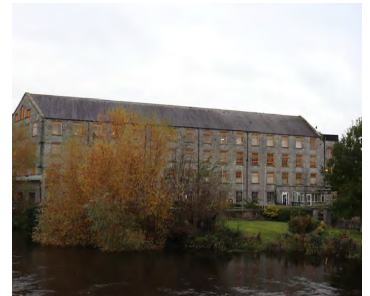
Celbridge Mill as it is today, vie from pedestrian bridge
