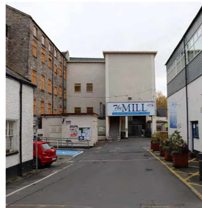
Entrance to Celbridge Mill community centre as it is today.
