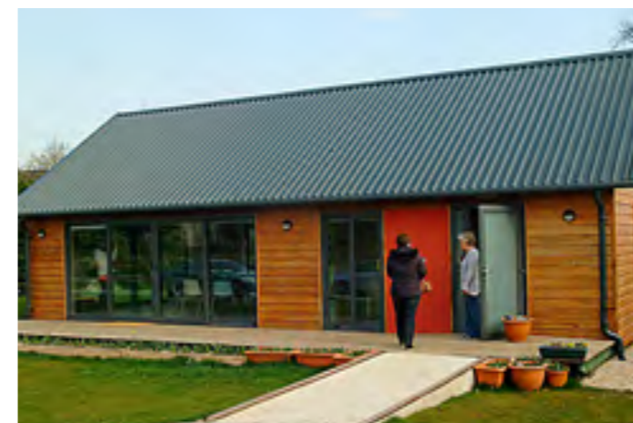
Acreproject.com. "Leader Application". Completed community building, June 2011
