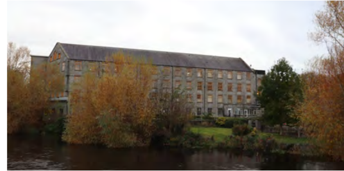
View of Mill building from pedestrian Bridge
