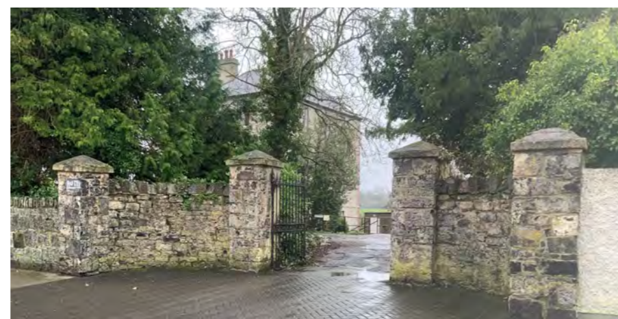
Parochial House Site Entrance from Main Street.
