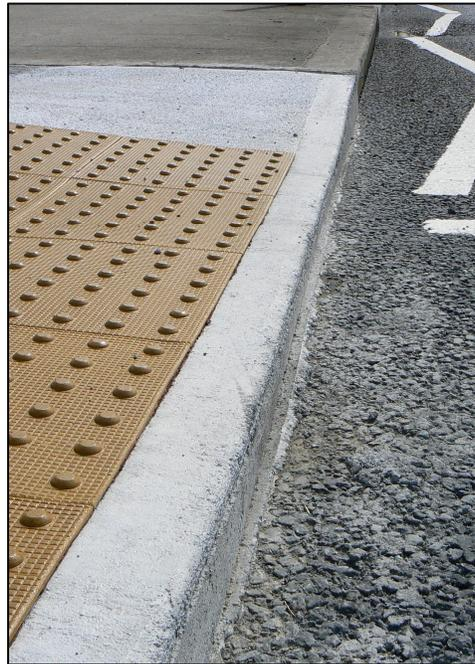
**Plate 9: 50mm upstand at new tactile crossing point, Scoil Na Mainistreach, Celbridge**
