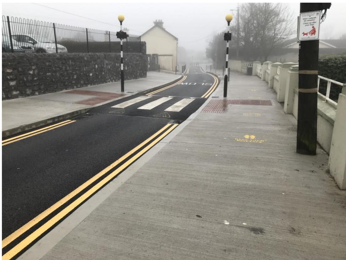
*Figure 6.12: Raised Table Zebra Crossing Recently Installed on Cleamore Road*
