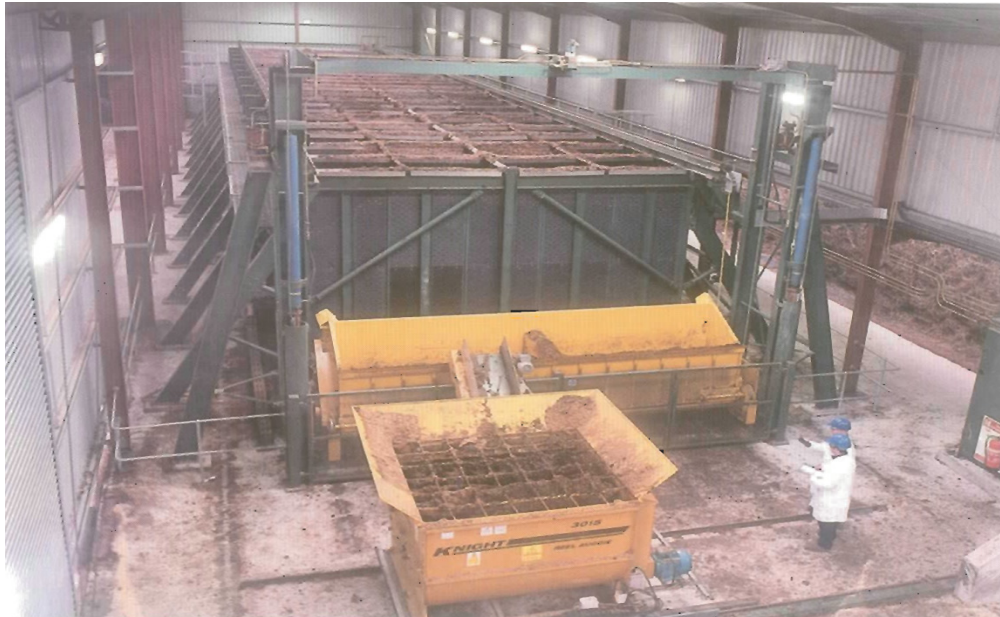
Figure 4.3: Sludge Treatment Facility at Silliot Hill (Source TEG)
