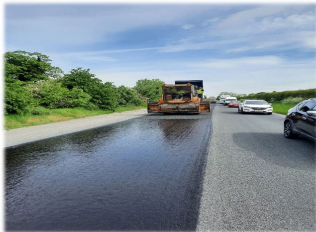
Surface dressing carried out by Kildare County Council transportation staff
