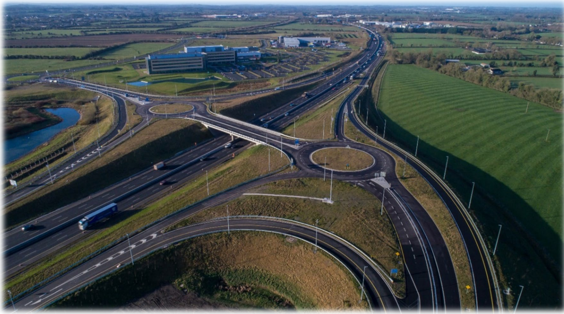
Aerial Photo – Junction 9a M7/Sallins Bypass
