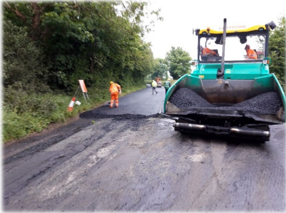
Restoration Improvement work carried out by contractor on site
