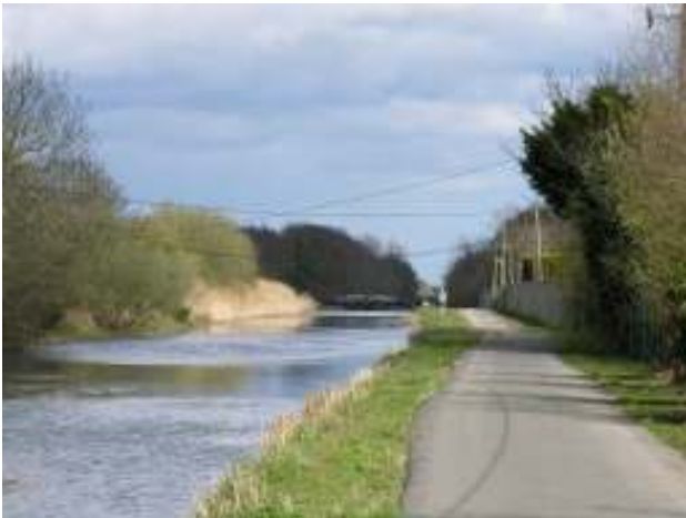
Figure 3: View along the Grand Canal Ardclough.
