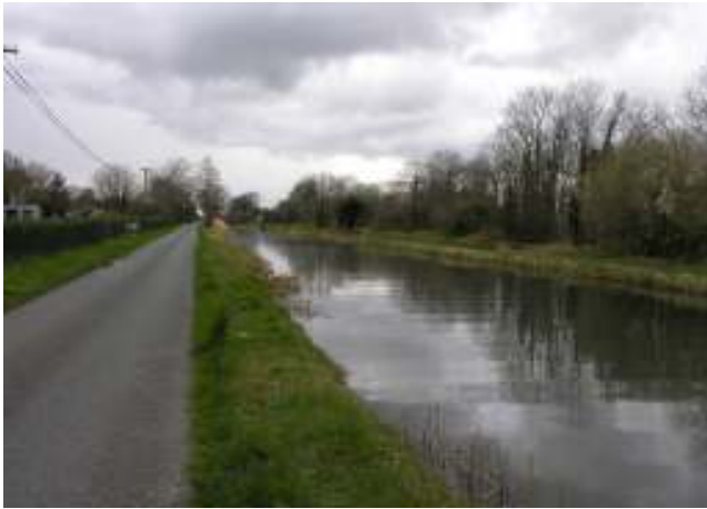
Figure 18: Lack of connectivity to the canal.
