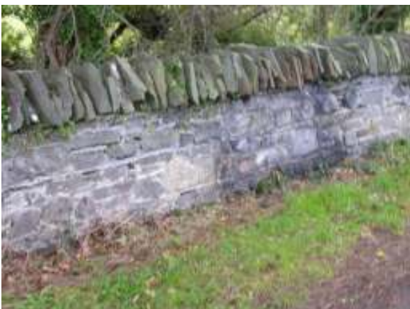
Figure 10: Restored stone wall.
