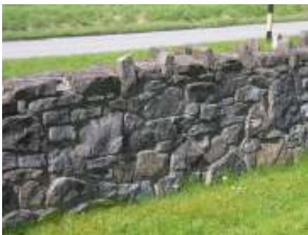
Figure 21: Stone walls to be retained.
