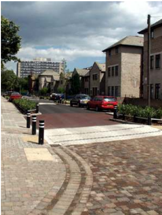
Figure 32: Above image is an example of the type of treatment of crossing points in the village, including a raised area for crossing and a clear demarcation of this pedestrian route using different coloured road surfacing and paving materials. Bollards and "pinch points" (in this case using planted areas) also act to calm and slow traffic.
