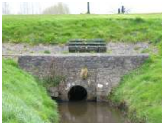
Figure 12: Single arch rubble stone aqueduct.
