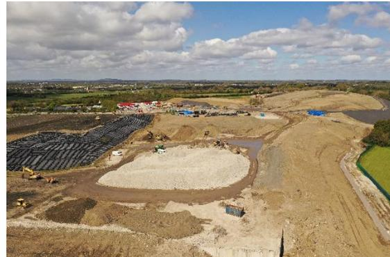
The contractor has already commenced the capping of the site with the Linear Low Density Polyethylene (LLDPE) sheeting.
